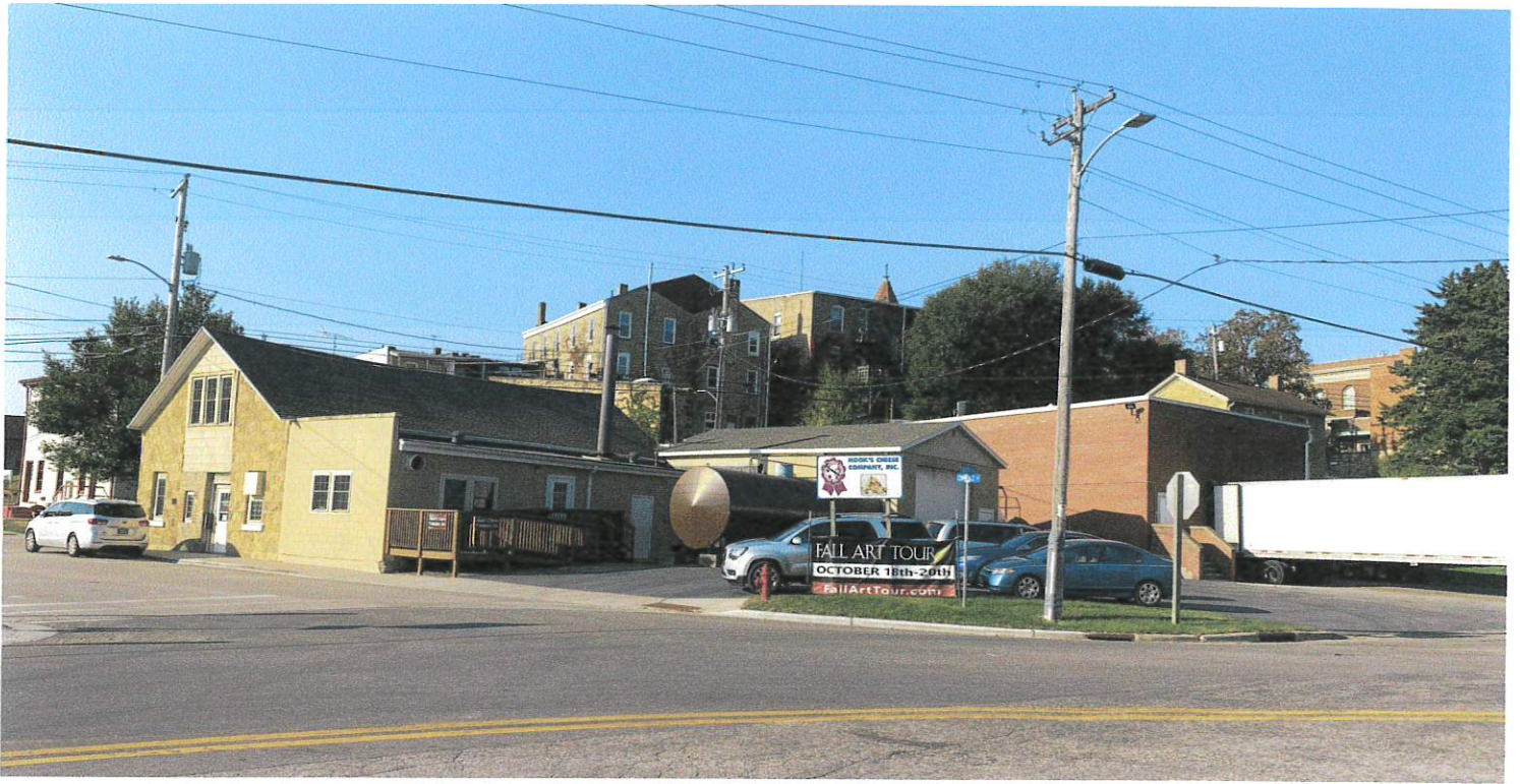
Exterior view from corner (Northeast)
