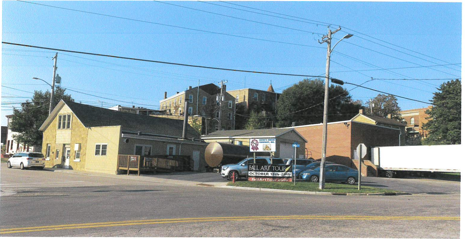
Exterior view from corner (Northeast)
