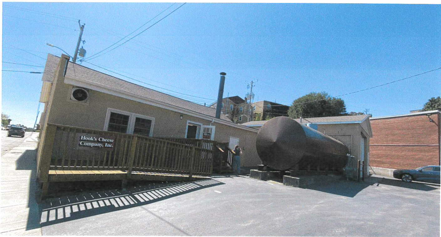
Store Entrance Exterior View (North)
