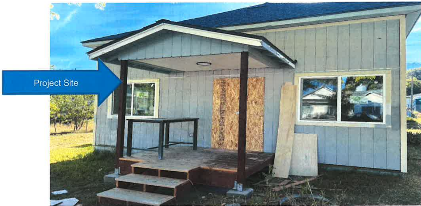
Figure 1 Site Location Front (Under Construction)
