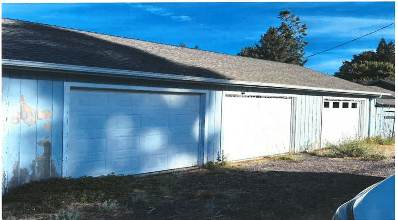
Figure 2 Site Location Rear
