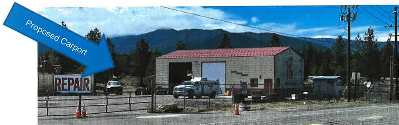
Figure 2 View of shop building and outdoor storage container. Proposed carport will be between the two
