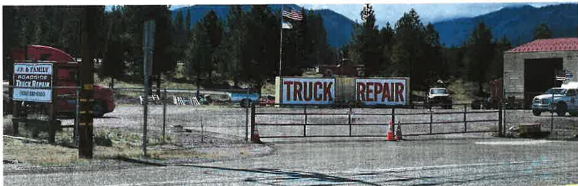
Figure 3 View of existing shop building and outdoor storage container
