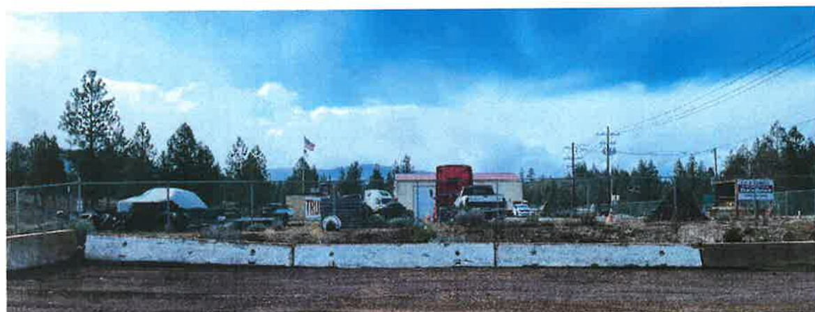
Figure 6 View north toward shop building showing outdoor storage of materials.
