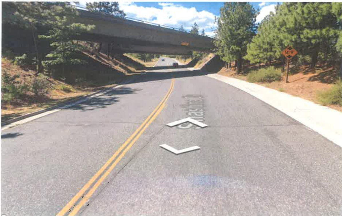
Figure 3 Street View Facing NW
