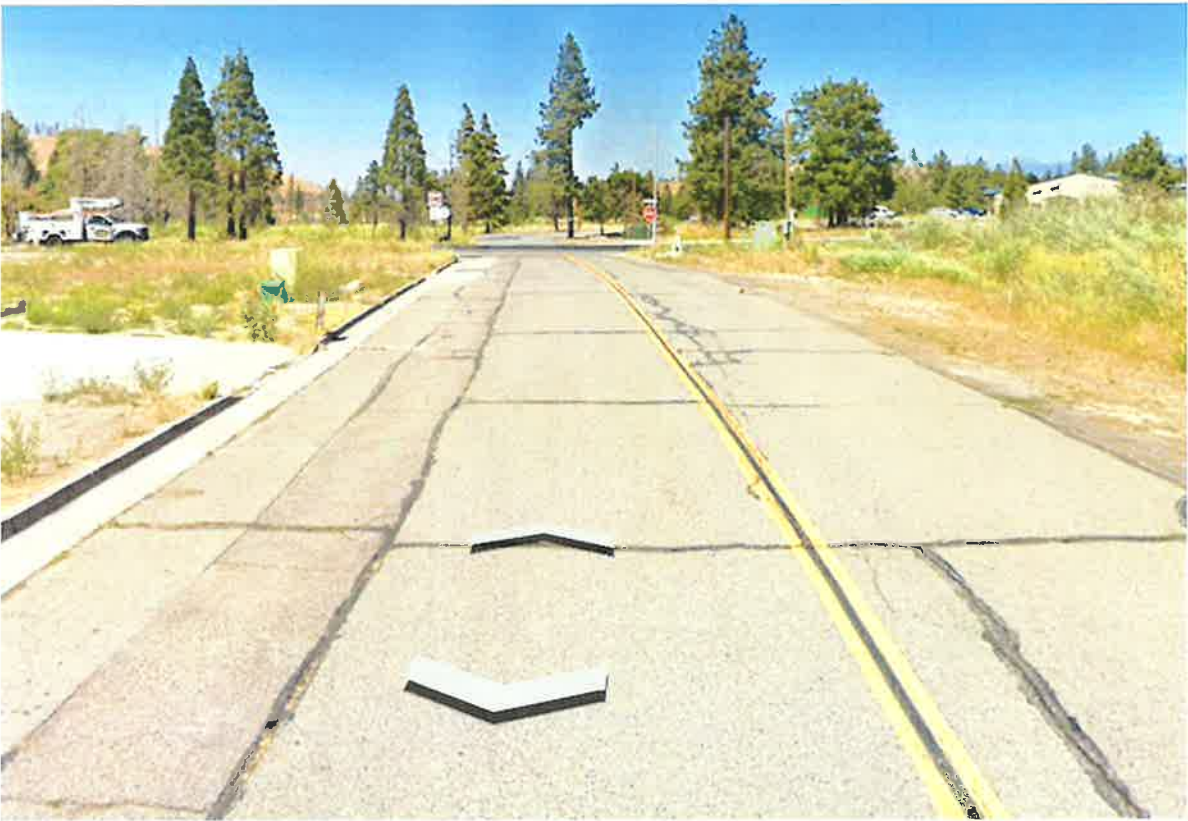
Figure 2 Street View North
