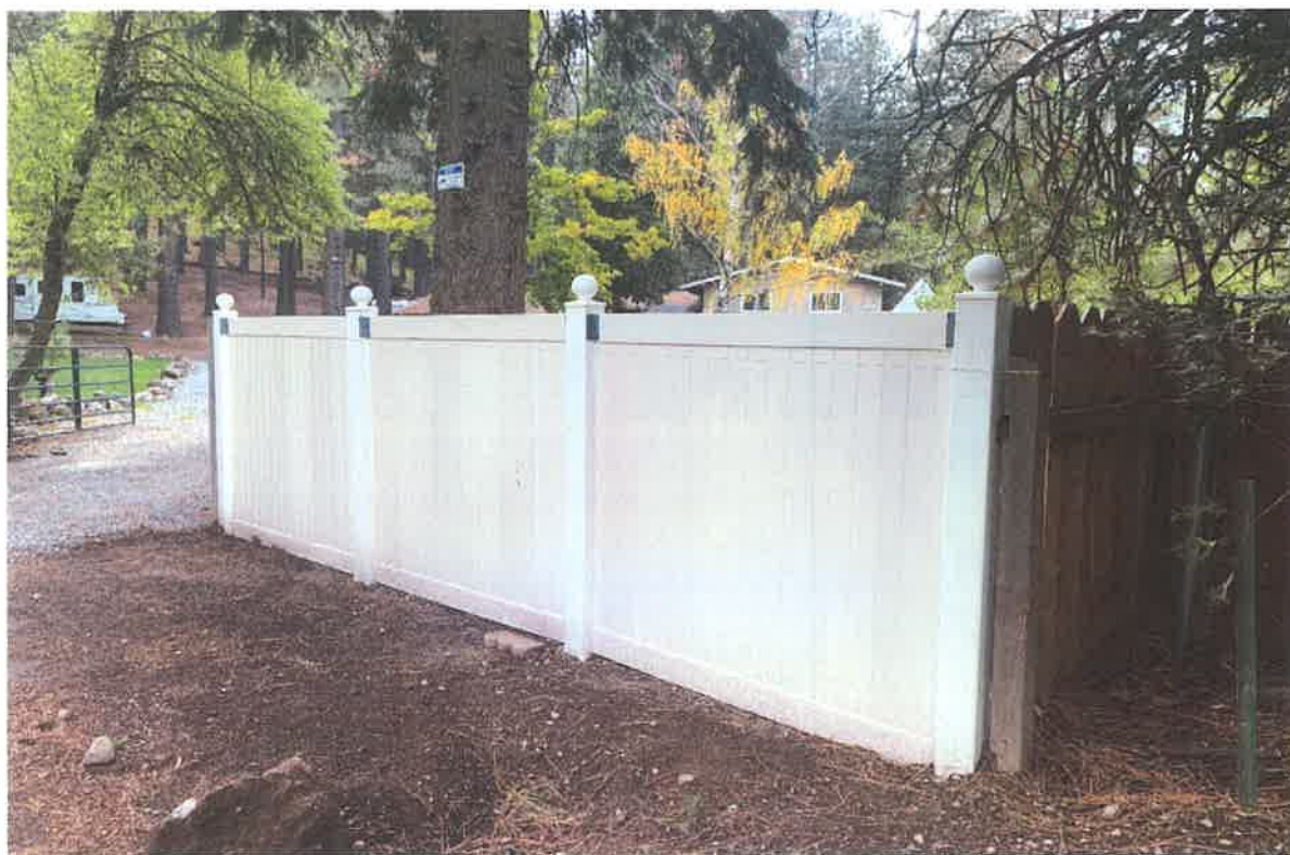
Figure 2 Solid Fence being constructed
