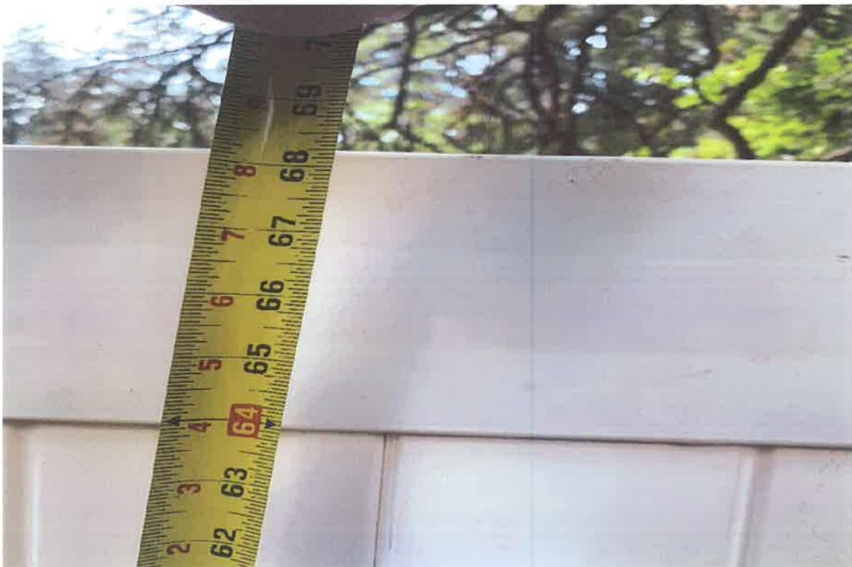
Figure 4 Height of fence previously constructed.
