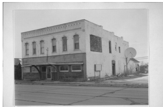
CA 110 S Division St. – Commercial Vernacular retail building; all or part of this building was built prior to 1894
