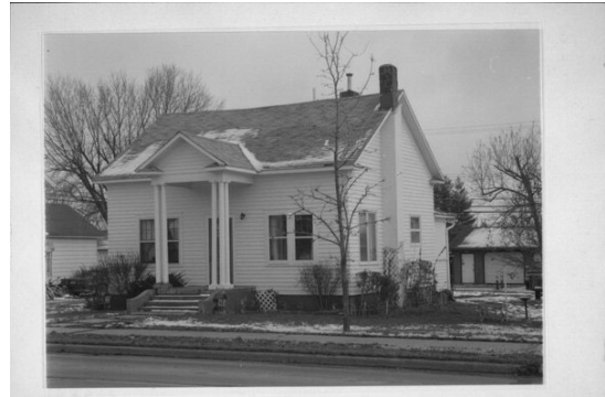
306 S Division St. – Side-gabled-style house
