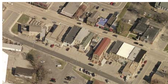
Spring Water Alley- existing condition
