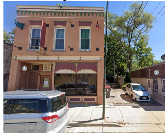
Image of Structure
