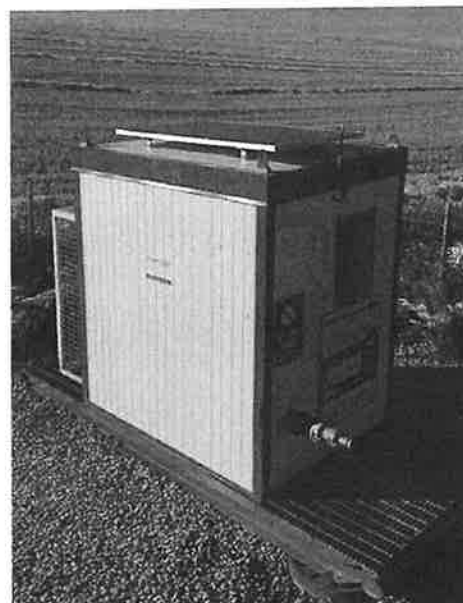
Portable, solar powered hydrant fill station with cellular communications and propane heater
