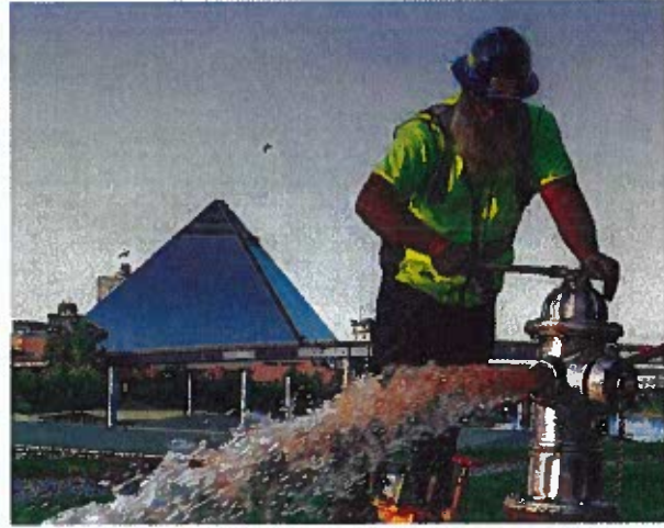
Hydrant Flushing in City of Memphis
