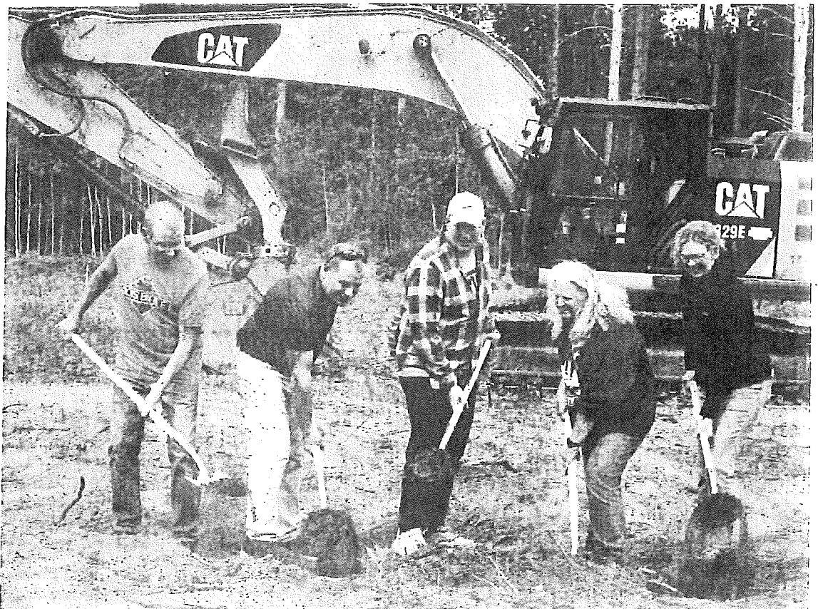
The board members symbolically break ground on the Town of Brule Garage construction project. Pictured, left to right: Kevin Mackie, Fred Stoll, Adam Olson, Jr., Diane Nelson and Amy Eliot.
