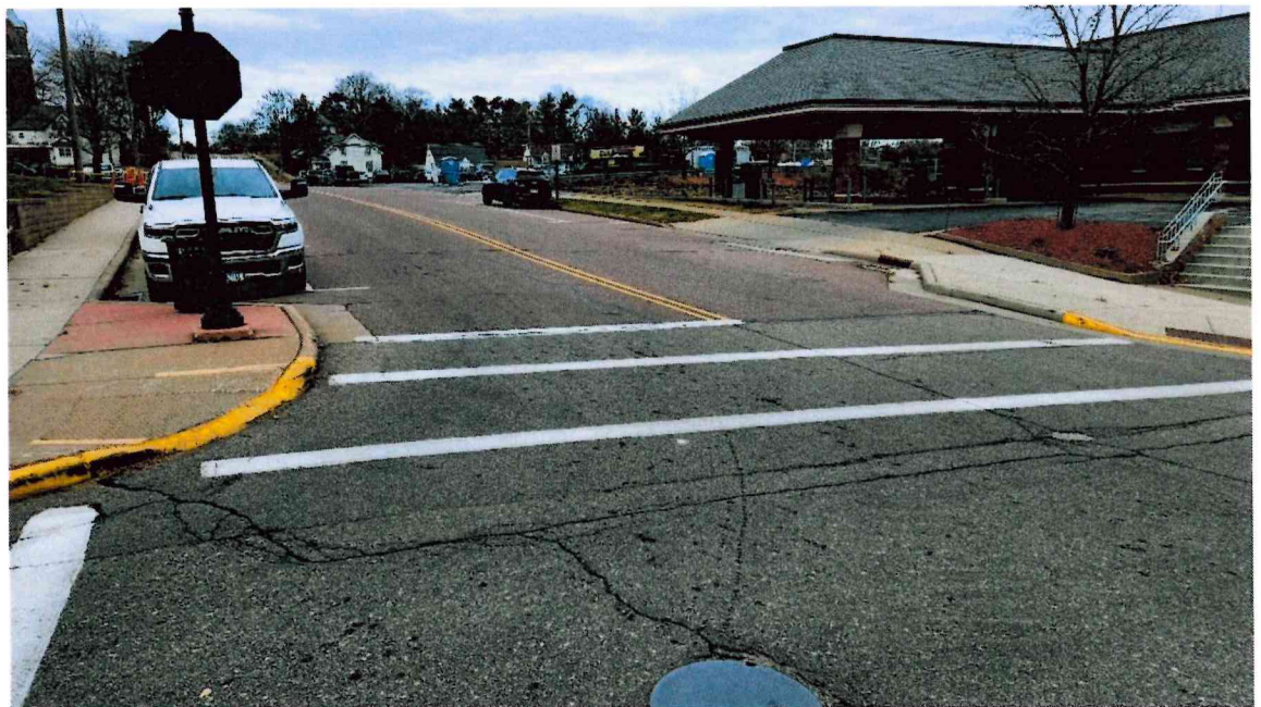
Figure 3 – Crosswalk at South End of Block (Looking North)
