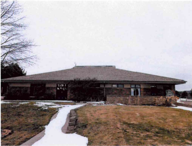
Photo of south roof face
