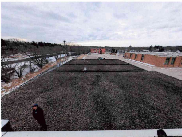
Photo of building from roof
