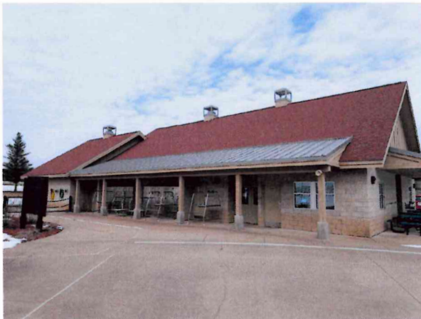
Photo of south facing roof
