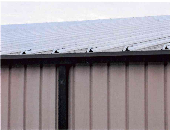
Photo of roof membrane
