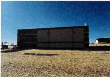
Wellhouse #3 East Elevation
