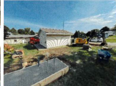
Wellhouse #2 Site Work
