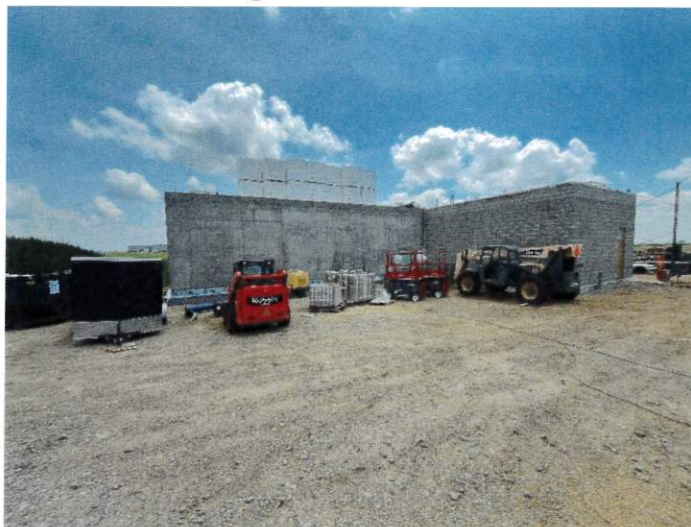
Wellhouse #3: July 15 th , 2025
