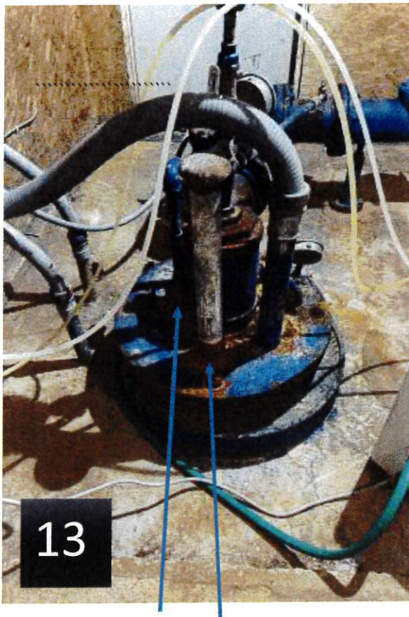
Well 2 vents (3/4 and 2") with 10" DIA borehole. Not sure if either pipe is > 24" off floor. Smaller DIA vent does not have a reverse bend or mushroom cap.
