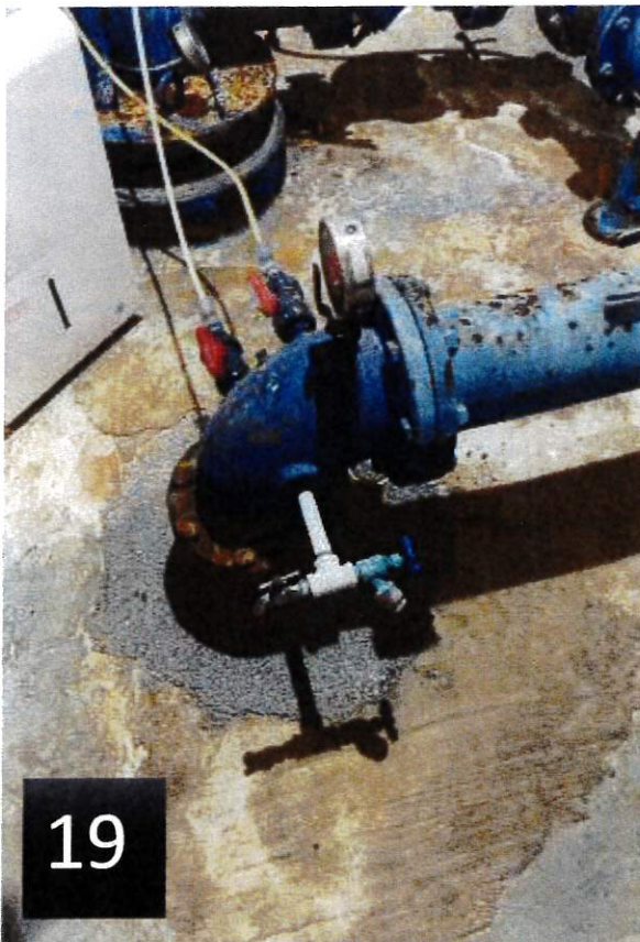
Well 2 sodium hypochlorite and fluoride injection point and nonconforming EP tap
