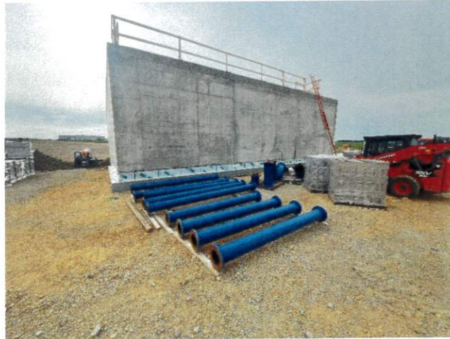
Ground Reservoir + Piping: April 2025
