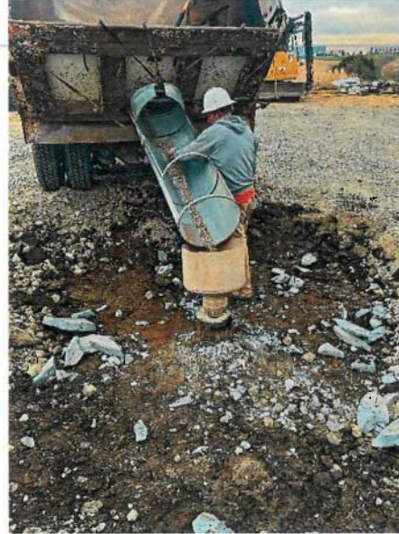
Sam's Well Drilling: Test Well Abandonment
