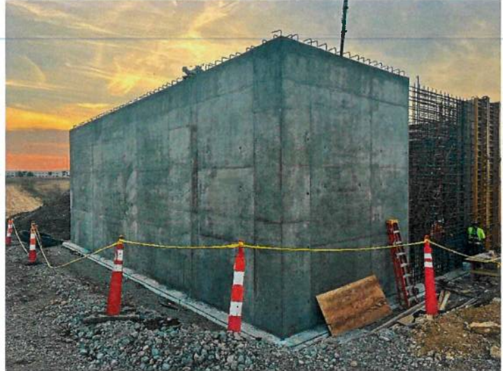
WELLHOUSE #3 FACILITY, RESERVOIR CONSTRUCTION
