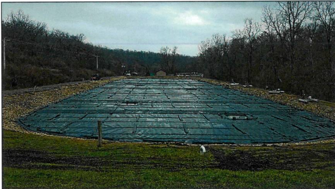
Figure 3. New lagoon cover and baffles in 2016 – 2017
