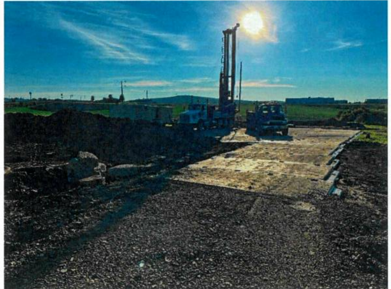
Sam's Well Drilling Rig at Final Well #3 Site
