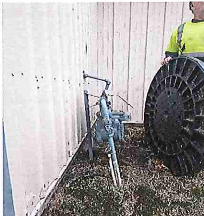
PUBLIC WORKS VENT LEAKAGE & UNPROTECTED UTILITIES.
