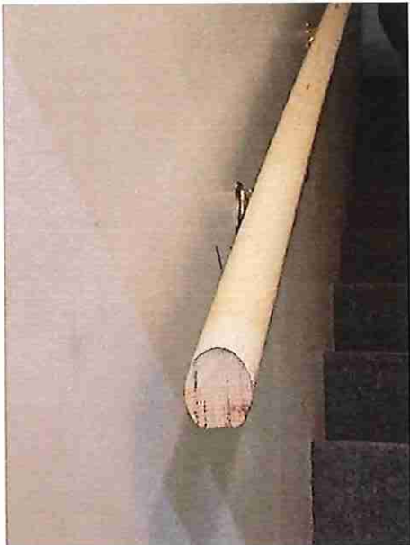
FIRE STATION NON-COMPLIANT HANDRAIL, REAR EXIT DOOR, & DOOR STOPS.
