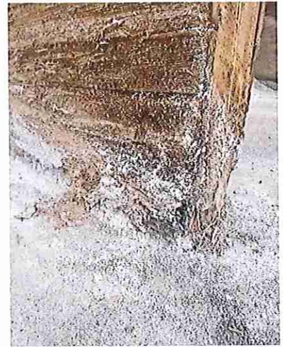
PUBLIC WORKS SALT STORAGE BUILDING DETERIORATION.
