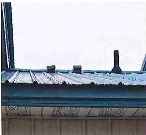
PUBLIC WORKS VENT LEAKAGE & UNPROTECTED UTILITIES.
