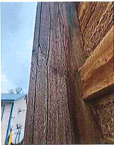
PUBLIC WORKS SALT STORAGE BUILDING DETERIORATION.
