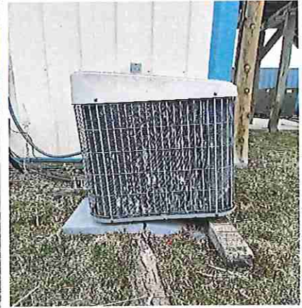
PUBLIC WORKS VENT LEAKAGE & UNPROTECTED UTILITIES.
