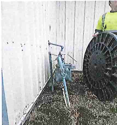
PUBLIC WORKS VENT LEAKAGE & UNPROTECTED UTILITIES.
