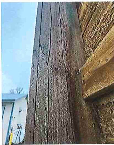
PUBLIC WORKS SALT STORAGE BUILDING DETERIORATION.
