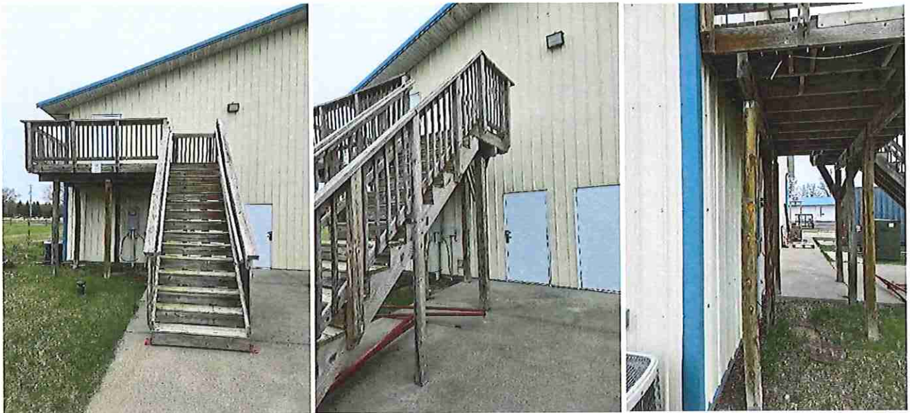
FIRE STATION REAR COMBUSTIBLE DECK.
