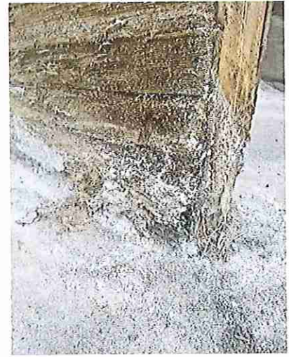
PUBLIC WORKS SALT STORAGE BUILDING DETERIORATION.
