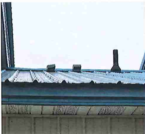
PUBLIC WORKS VENT LEAKAGE & UNPROTECTED UTILITIES.
