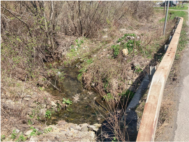
Photo 51: ETWB on 4/15/24. View from Rte. 44 facing East.
