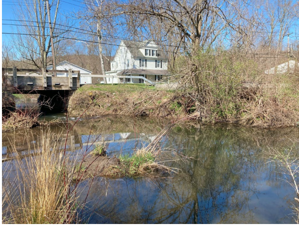
Photo 9: ETEBUSMS and downstream on 4/15/24, view of Mechanic Street bridge
