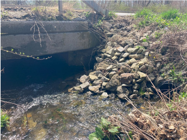
Photo 52: ETWB on 4/15/24. Downstream view. Outfall visible bottom right.
