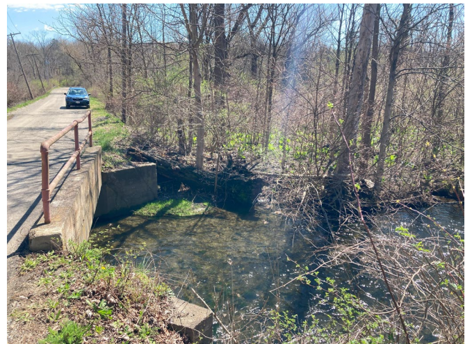
Photo 47: ETDSLB on 4/15/24, facing East
